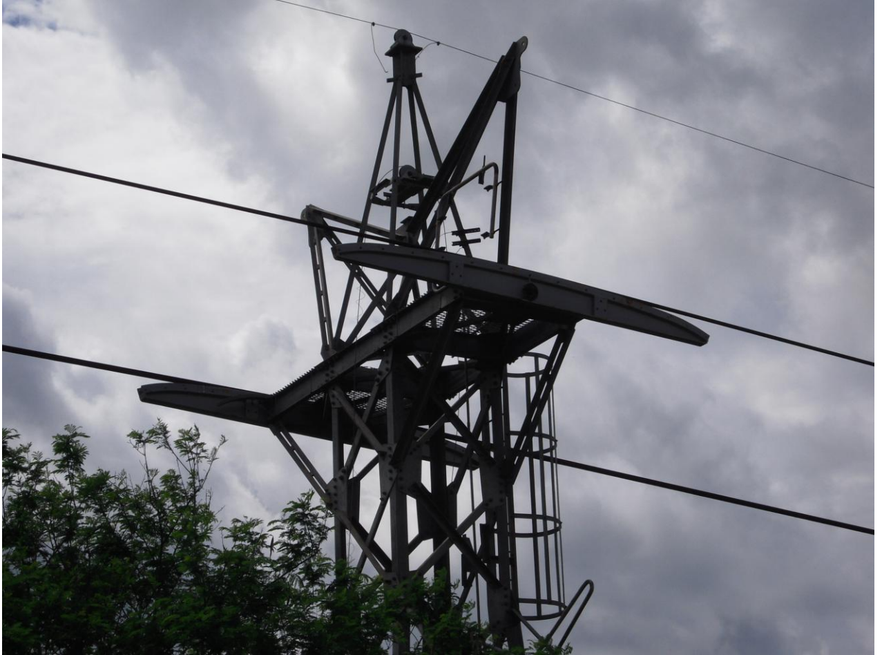
Typical tower of a ropeway with oscillating saddles.
